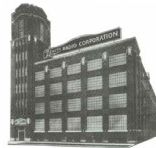
In 1924, burgeoning Zenith moved to this factory at 3620 Iron Street.
